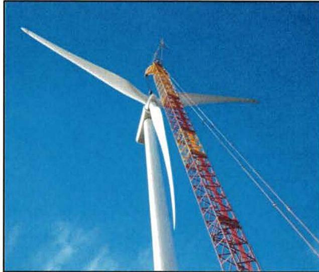
Figure 1.1-1. Example wind turbine.
