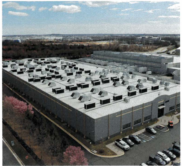
Another data center in Ashburn, Virginia.
