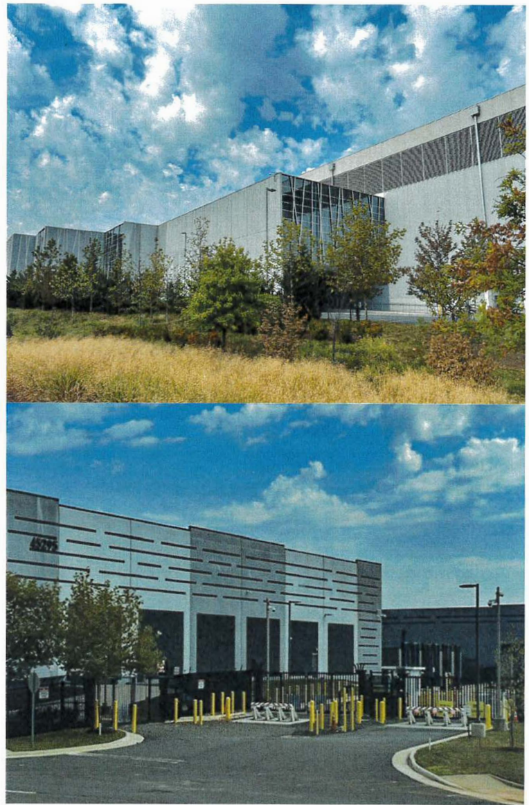
Two examples of data centers located in Ashburn, Loudoun County, Virginia.
