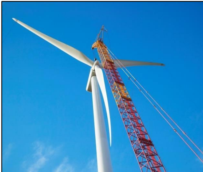
Figure 1.1-1. Example wind turbine.
