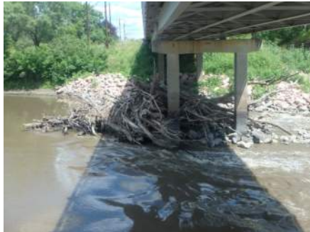
Tree Debris at Bent 5
