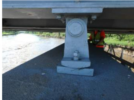
Typical Bearing at Bent 3
