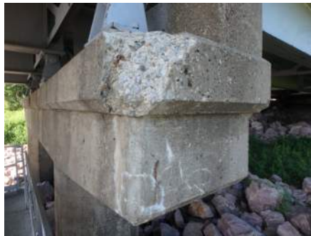
Concrete Deterioration on the North End of Bent Cap 2
