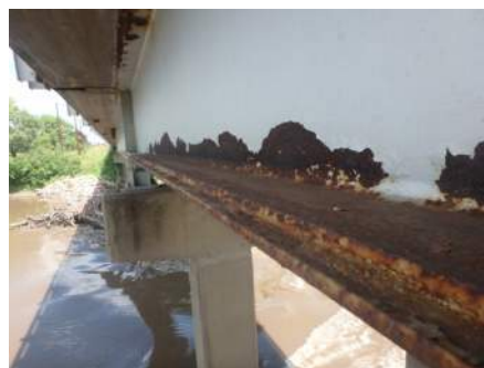
Typical Corrosion to the Exterior Girders
