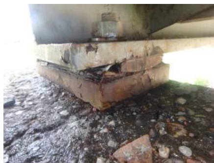
Section Loss of Bearing Plate over Bent 2
