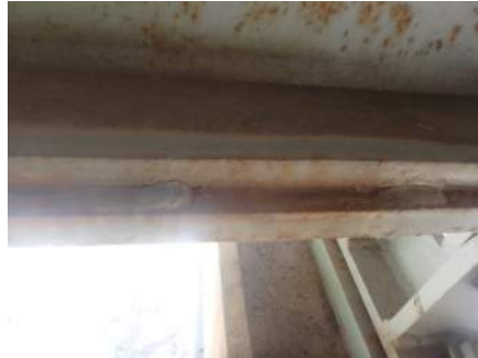
Cracked Weld on Girder 3 over Bent 5 on the Cover Plate
