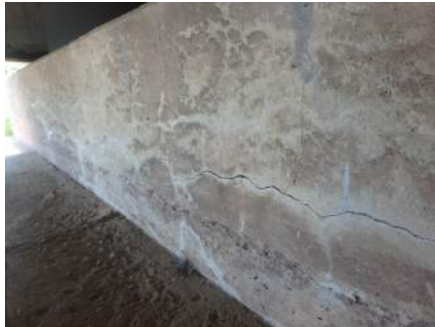
Cracking on Abutment 1 Sill
