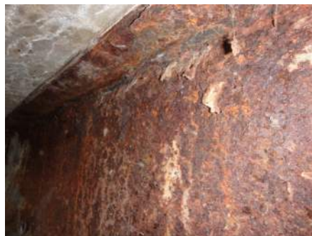
Typical Section Loss to the Web of the Girders
