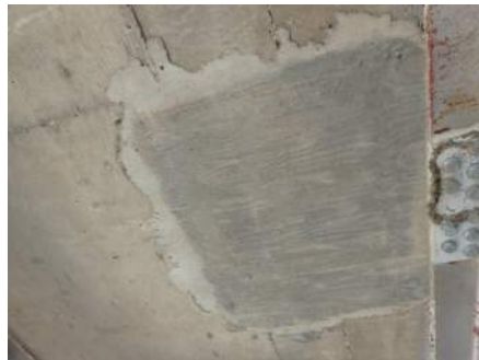
Concrete Patching on the Underside of the Deck at Bolted Splice Locations
