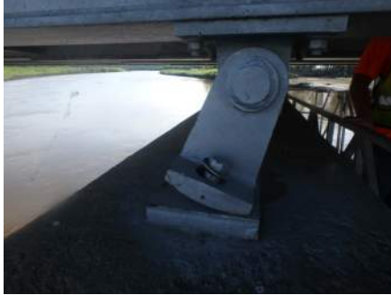
Typical Bearing at Bent 3
