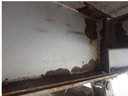
Corrosion of Girders over the Bents
