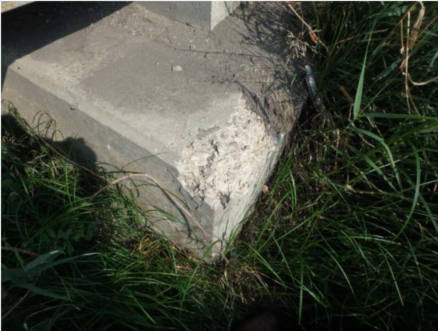
Concrete Deterioration on the East End of Abutment 6
