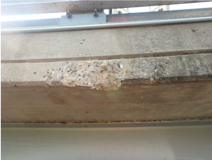
Spall on the North Side of the Deck near Bent 6
