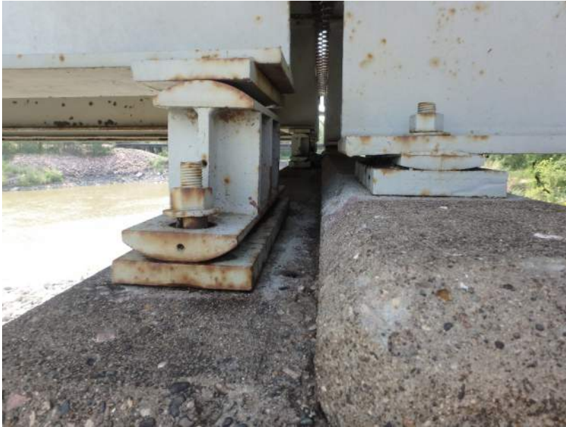
Typical Bearings at Bent 3
