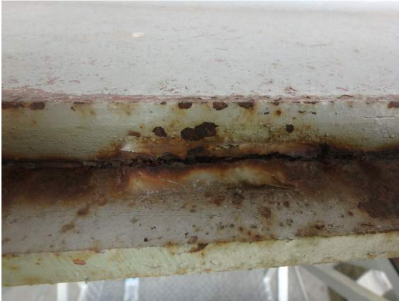
Broken Weld on Girder 4 in Span 2 on the Outside of the Cover Plate (Typical to numerous locations)
