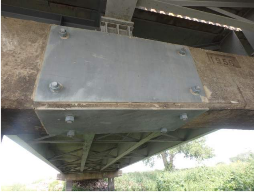
Bent Cap Repair on Bent 5
