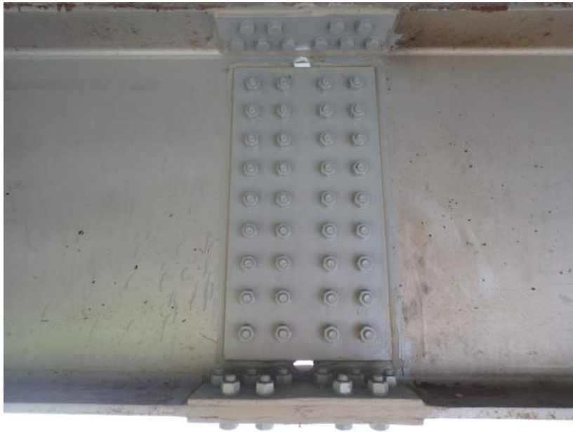
Typical Bolted Splice
