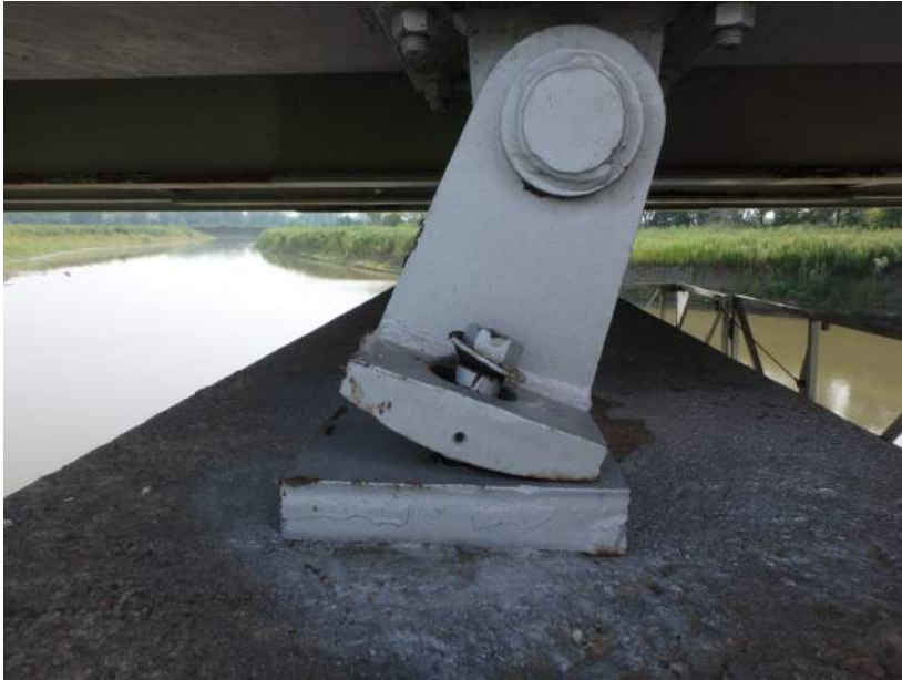
Typical Rocker Bearing at Bent 3
