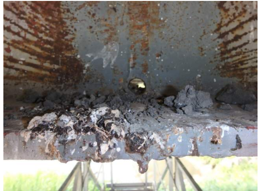
Hole in Web of Girder 2 in Span 2 near Bent 3
