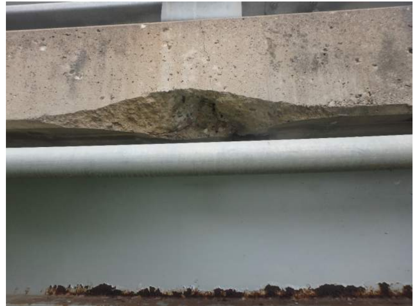
Spall on the South Overhang in Span 1
