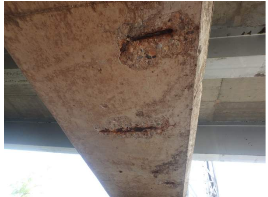
Exposed Rebar on the Underside of Bent Cap 2
