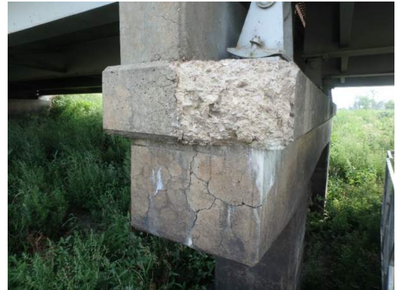
Concrete Deterioration on the West End of Bent Cap 5
