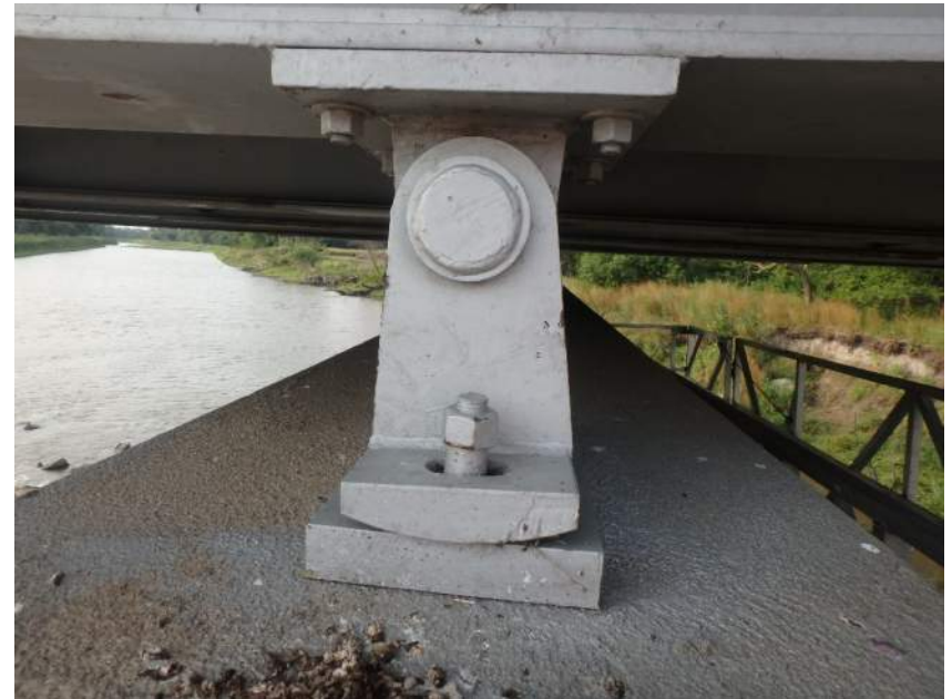
Typical Bearing at Bent 3
