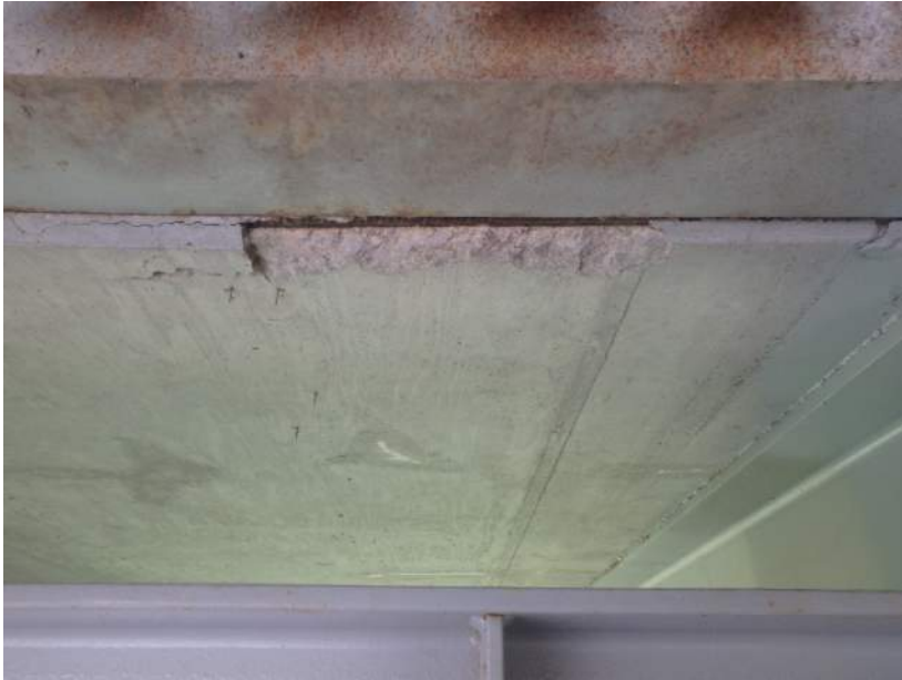
Spall with Exposed Rebar in Bay 1 over Bent 5
