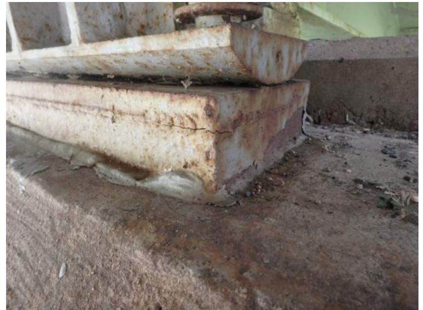
Cracked Bearing Plate at Bearing 2 Bent 2 North Side
