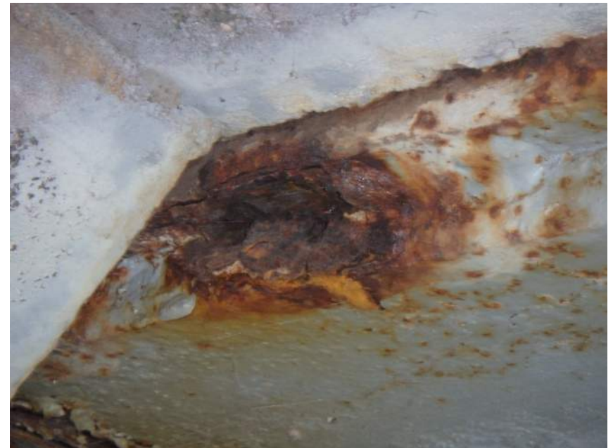
Broken Weld on Girder 4 at Bent 6 on Top Flange
