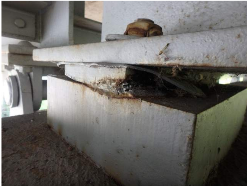
Typical Pack Rust on Bearings 2 & 3 at Bent 2 in Span 1
