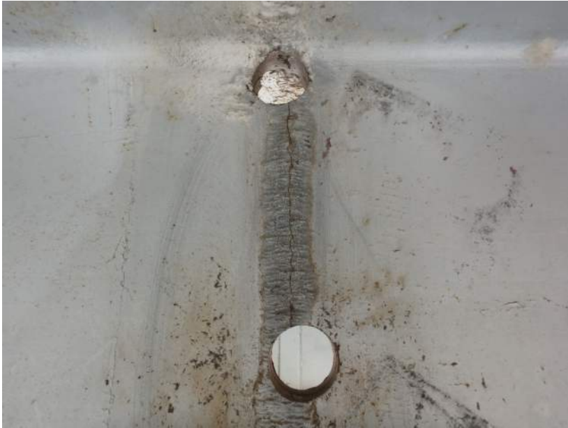
Arrested Crack on Girder 2 Span 3
