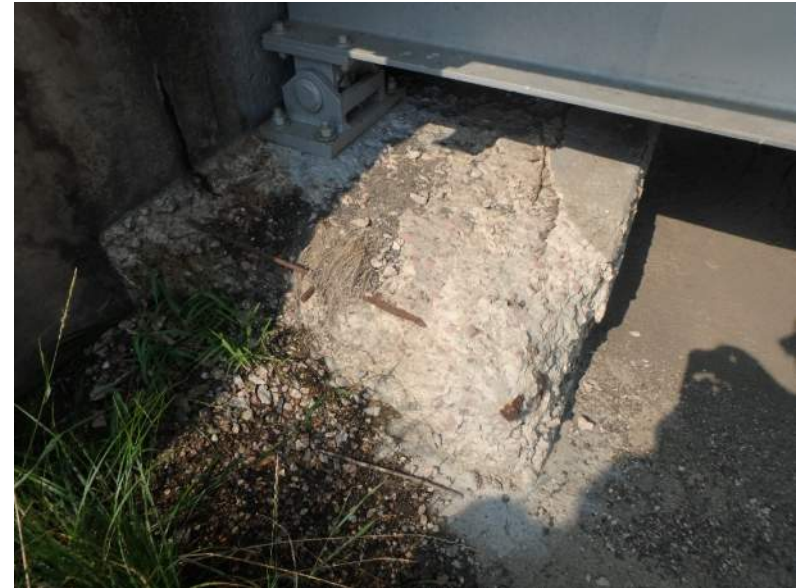
Severe Concrete Deterioration with Exposed Rebar on the East End of Abutment 1
