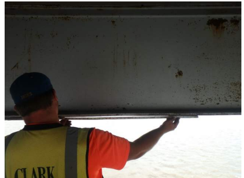
Bent Girder at End of Cover Plate in Span 3
