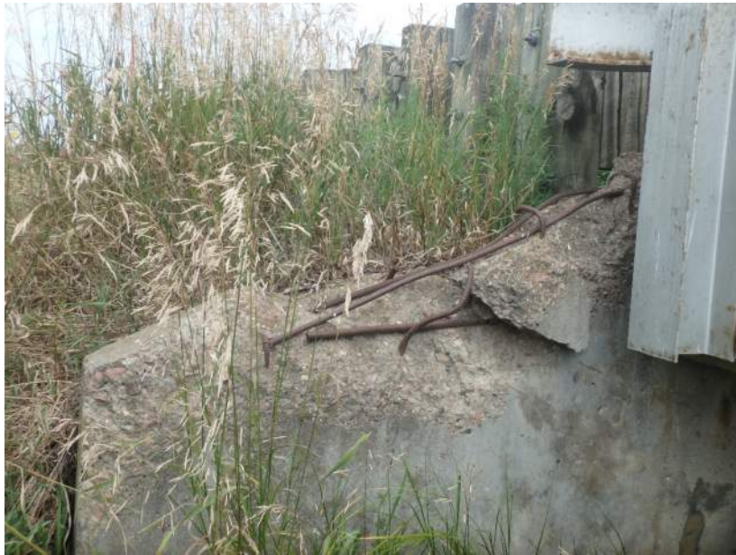
Collision Damage with Exposed Rebar on the Northeast Wingwall
