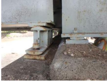
Typical Bearings at Bent 3
