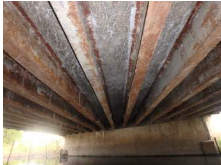
Typical Underside of the Deck and Girders
