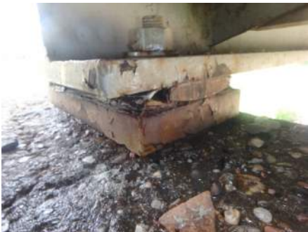
Section Loss of Bearing Plate over Bent 2
