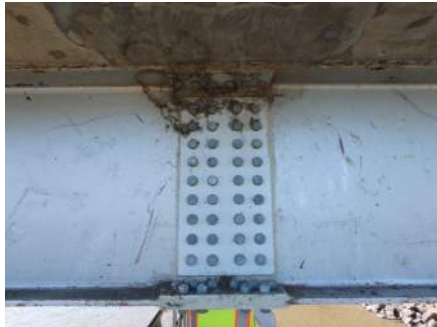
Typical Bolted Splice Plate
