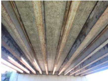
General Layout of the Underside of the Deck and Girders
