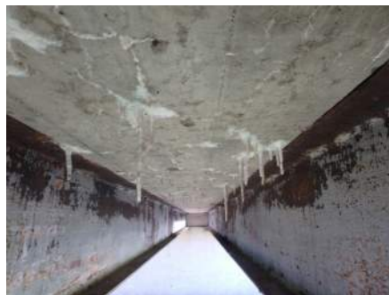
Typical Stalactites Buildup on the Underside of the Deck
