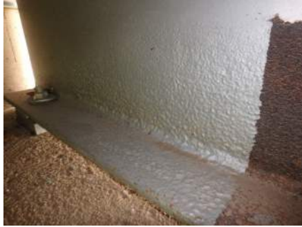
Typical Painted Ends of Girders
