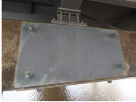
Bent Cap Repair on Bent 5
