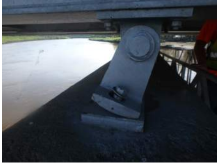
Typical Bearing at Bent 3
