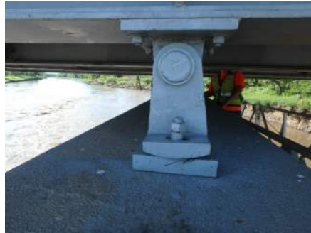
Typical Bearing at Bent 3
