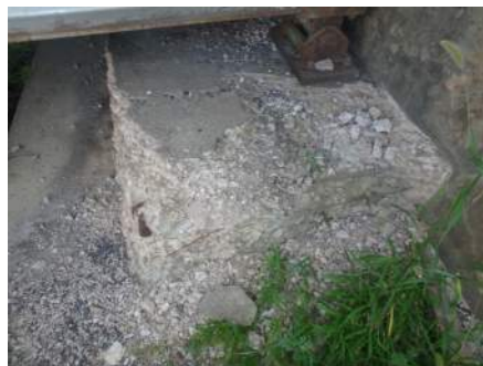
West End of Abutment 1
