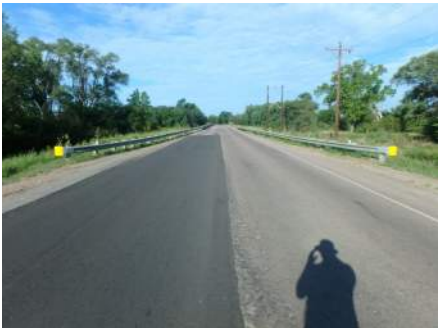
Alignment Facing West
