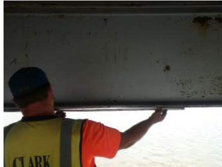
Bent Girder 3 at End of Cover Plate in Span 3
