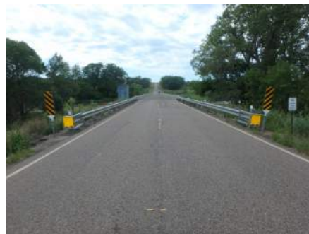
Alignment Facing West
