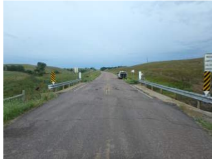
Alignment Facing West
