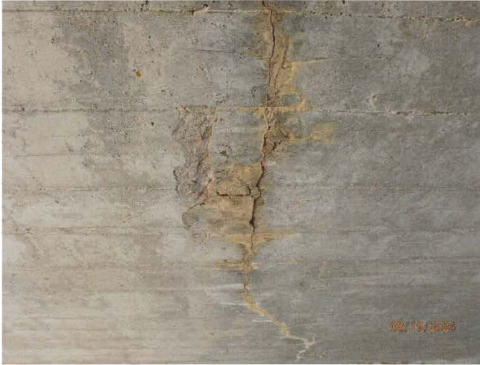
Delamination near Midspan of Span 1
